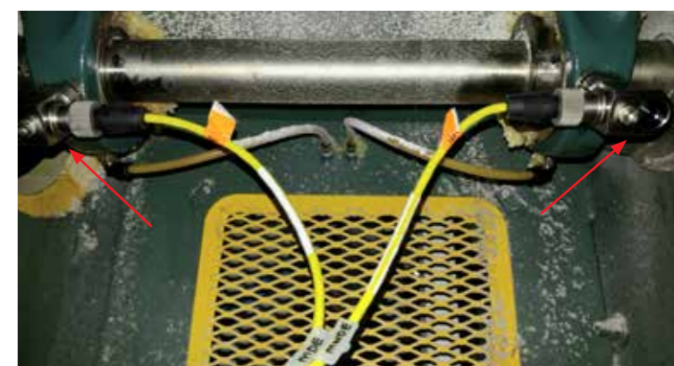
The vibration sensors were successfully installed in the running motor systems
